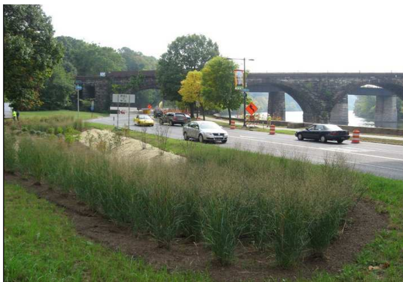
Figure 1 Vegetated Swale, Philadelphia, PA (USEPA, picasaweb)
