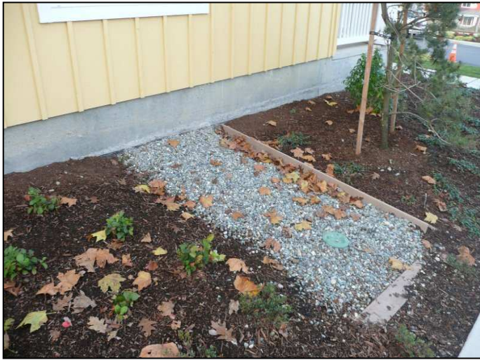
Figure 1 Infiltration Bed, Seattle, WA (USEPA, picasaweb)
