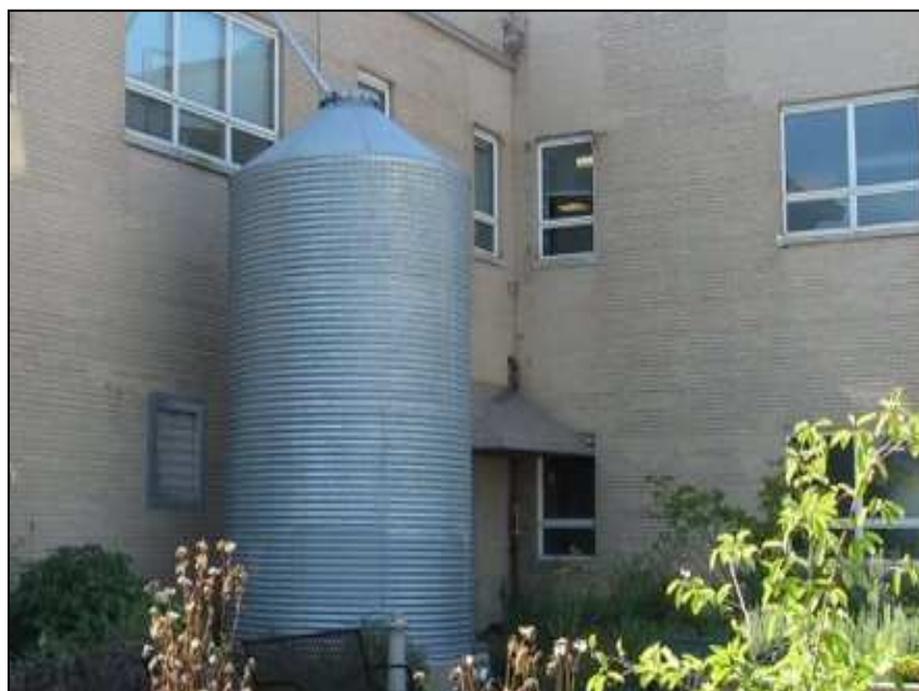
Figure 1 Above ground cistern, Chicago, IL (USEPA, picasaweb)
