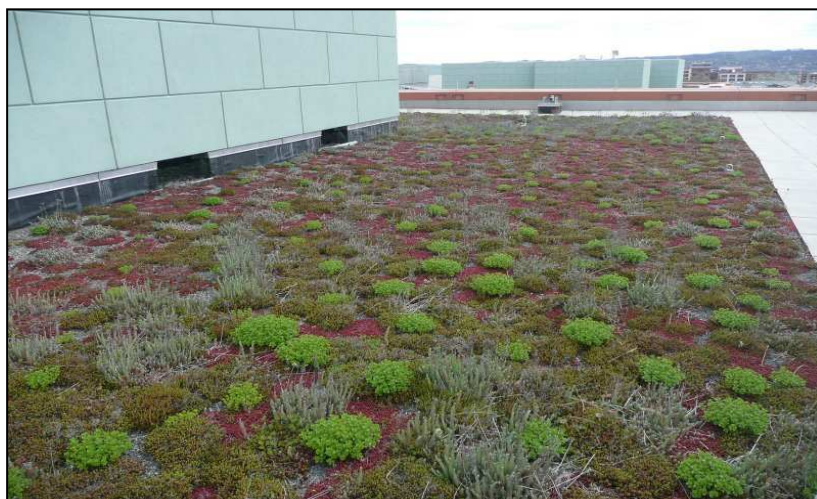
Figure 1 Vegetated Roof, Washington, DC (USEPA, picasaweb)
