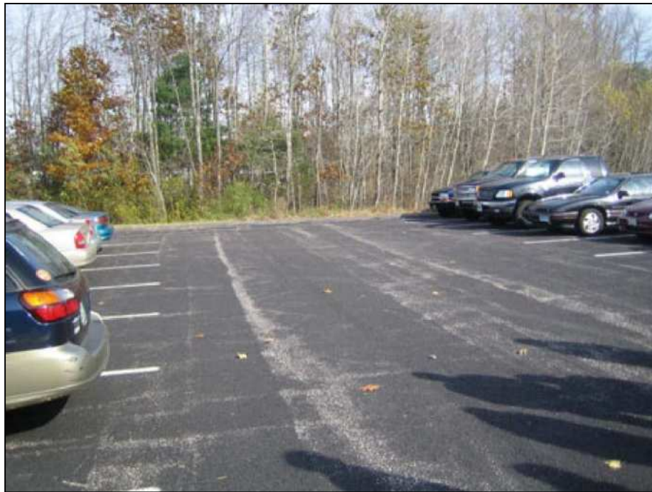
Figure 10.2.1 Example of a Porous Asphalt Parking Lot
